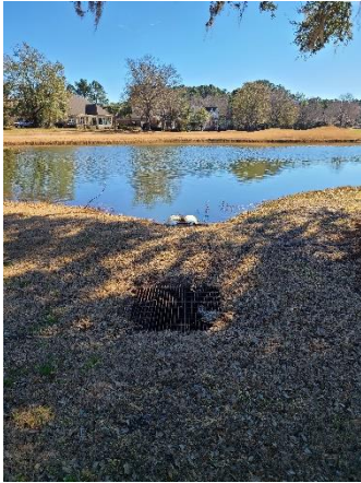
Photo 13 - Inlet 5 from Inlet 4 Looking Southeast
