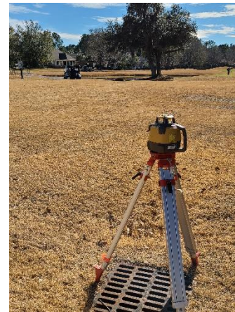
Photo 10 - Inlet 3 Looking Southeast (Downstream)
