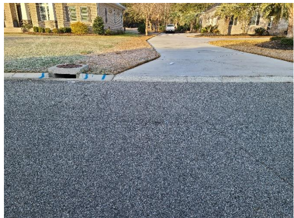
Photo 6 - Roadway Section (Inlet 1 in Background)
